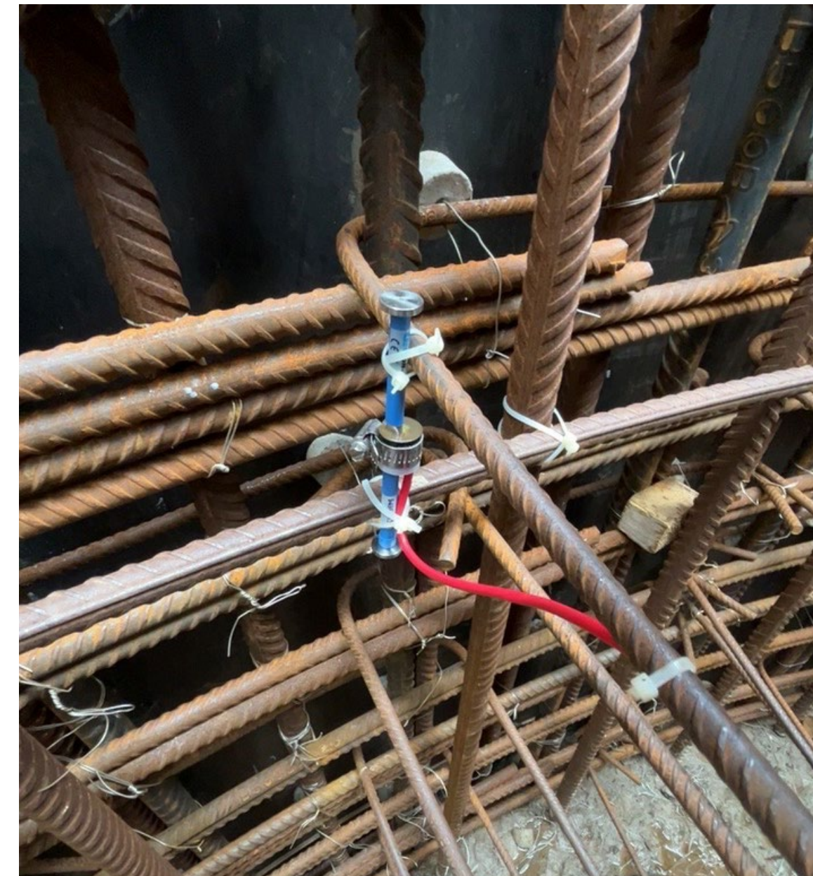
Pylon Strain gauge and thermistor
